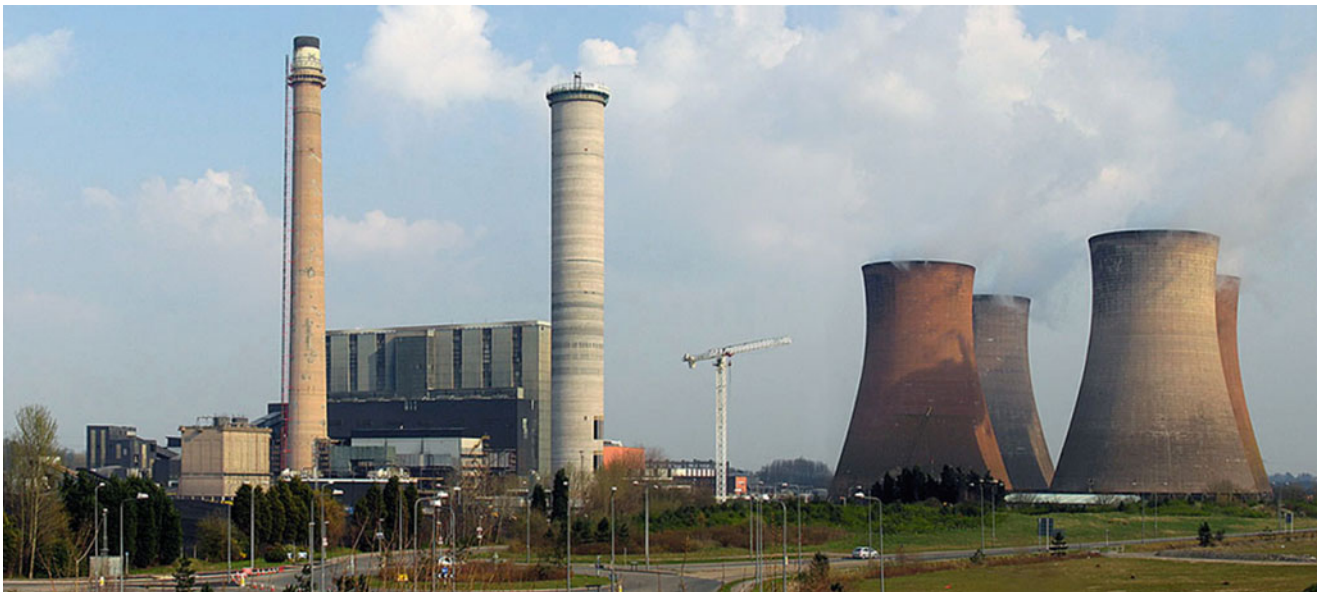
Fig. 22.4 Old (left) and new (right) chimney of the Rugeley Power Station
