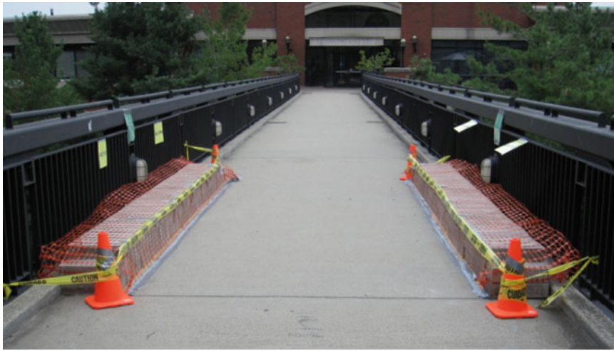
Fig. 5.4 Concrete blocks loaded on footbridge's deck for 3 days
