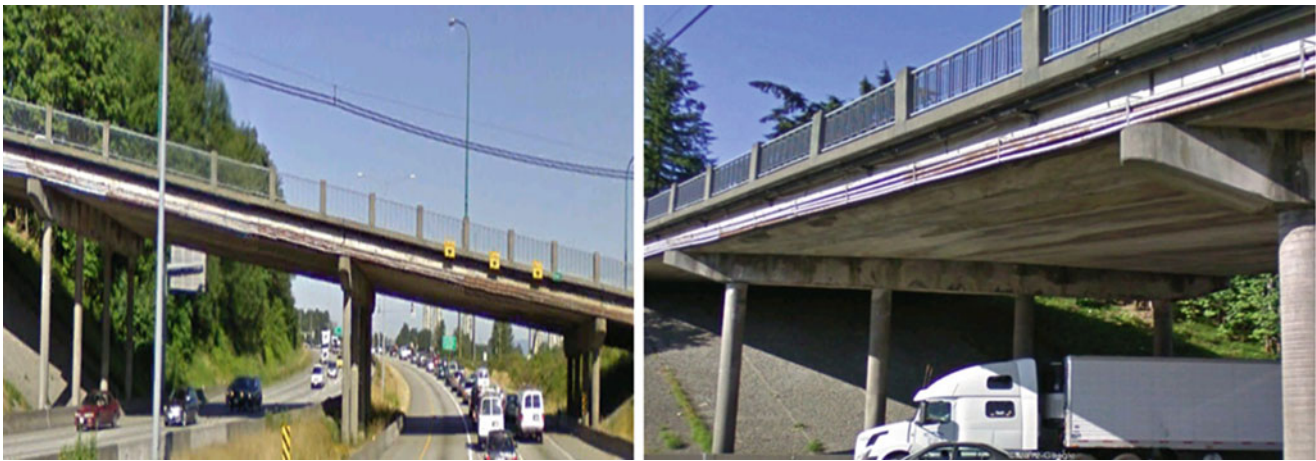
Fig. 15.5 Douglas road underpass (Douglas Rd)
