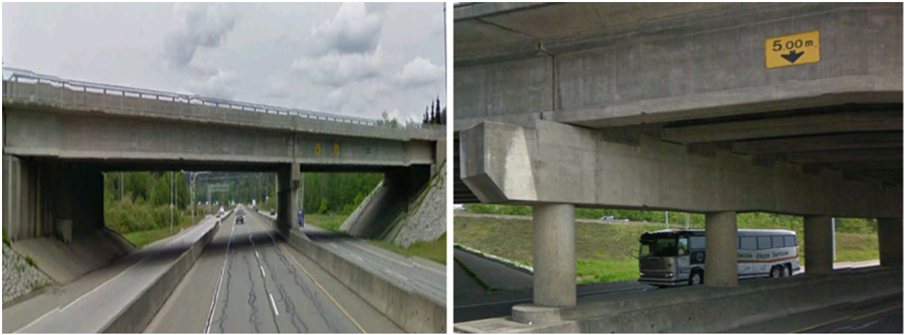
Fig. 15.3 Annacis highway and Highway 10 underpass (HWY 10th)
