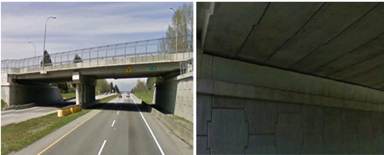
Fig. 15.2 Highway 99 and 24th avenue underpass (HWY 24th)
