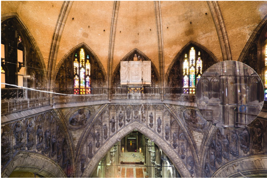
Fig. 16.5 Fiber optic sensors mounted on cupola of the Duomo di Milano
