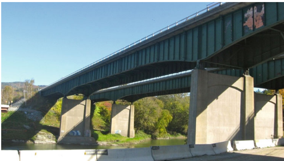
Fig. 12.1 Overall view of bridge 58 N in I-89 Vermont
