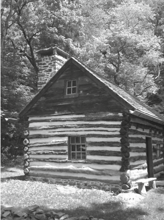
Fig. 9.4 The Lower Swedish Cabin located on Creek Road in Drexel Hill, Pennsylvania. This is one of the extant seventeenth-century cabins in the New Sweden area which have been attributed to the forest Finns due to its log construction (Jordan and Kaups 1989:151). (Photo by Ulla Isabel Zagal-Mach Wolfe)
