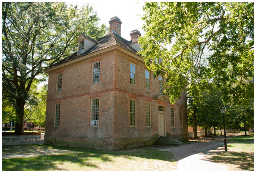
Fig. 17.1 Building of the Brufferton Indian School established in 1723 at the College of William and Mary in Williamsburg, Virginia. Photo courtesy of Mark Kostro, Colonial Williamsburg Foundation
