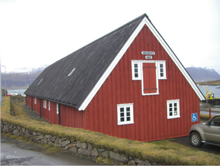
Fig. 3.4 The trading station of Djúpivogur (Photo by Gísli Pálsson)
