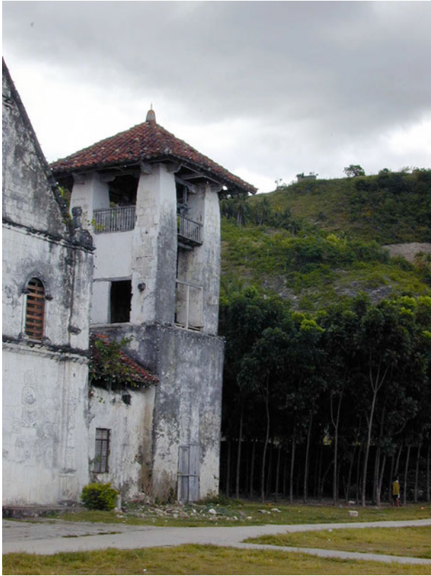
Fig. 4.3 Boljoon tower and baluarte on hill in background designed and built by Julian Bermejo
