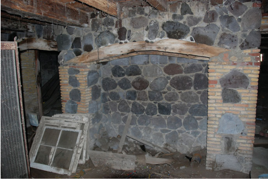
Fig. 3.2 The full cellar under a 1750s merchant's home in Oranjestad, St. Eustatius that exhibits the reuse of ship's rib as arch supports
