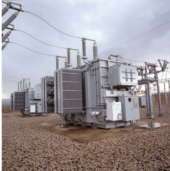
Fig. 2.26 Voltage transformers (Courtesy of General Electric)
