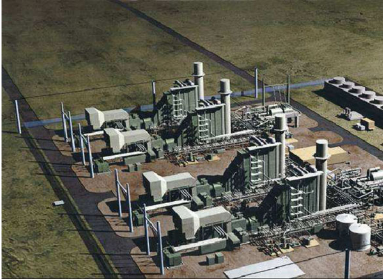
Fig. 15.18 Illustration of a 2×207FA (two Frame-7 60-Hz GTs with single ST) NG CC power plant. From left to right , for each GT-HRSG “block” one can see the GT inlet air filter housing and duct (on top of the GT enclosure), HRSG with drums on the top, and the stack. Two STs are located to the right of the GT-HRSG blocks (cross-over pipe and down-flow LP section are clearly visible). Note the elevation of the ST structure to accommodate the steam condenser. Partially visible to the right is the multicell mechanical cooling tower. In the lower right corner are two distillate oil (GT backup fuel) tanks (Courtesy: GE Energy)
