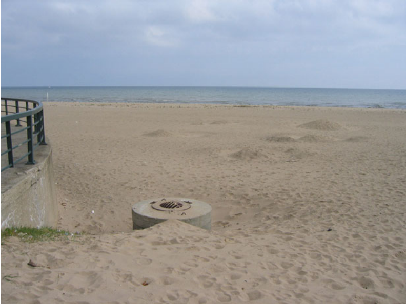
Fig. 9.3 Stormwater outfalls introduce fecal pollution from domestic pets and wildlife into rivers. Stormwater systems can also become contaminated with human sewage from leaking sanitary sewer systems (Photos provided by Dr. Sandra McLellan, University of Wisconsin-Milwaukee)
