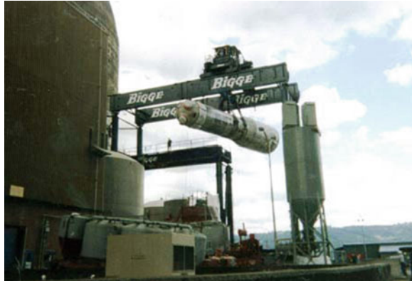
Fig. 9.4 A steam generator is removed from a reactor building [76]
