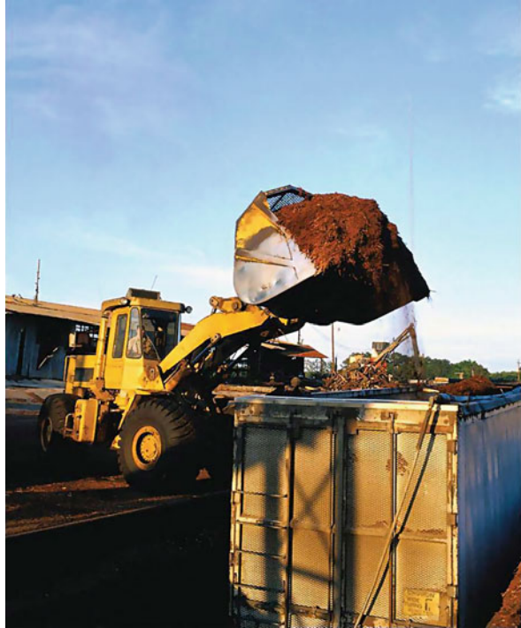
Fig. 9.7 Removing uncontaminated soil and debris for offsite disposal [42]
