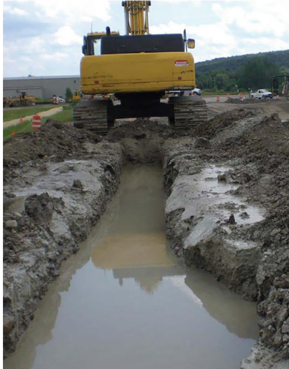
Fig. 9.8 Building a slurry wall to remediate contaminated groundwater [42]
