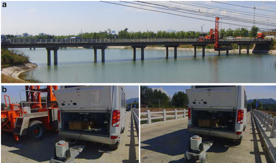
Fig. 14 The Chao He Bridge (a) elevation (b) on-site inspection
