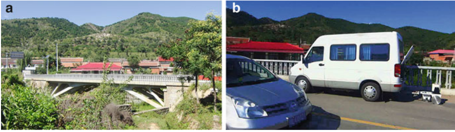
Fig. 11 The Hong Shi Kan Bridge (a) elevation (b) on-site inspection
