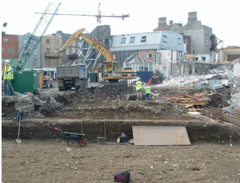
Illus. 12.1 Archaeological excavation (foreground) as part of the construction/demolition process on a site in Dublin city centre (Linzi Simpson)
