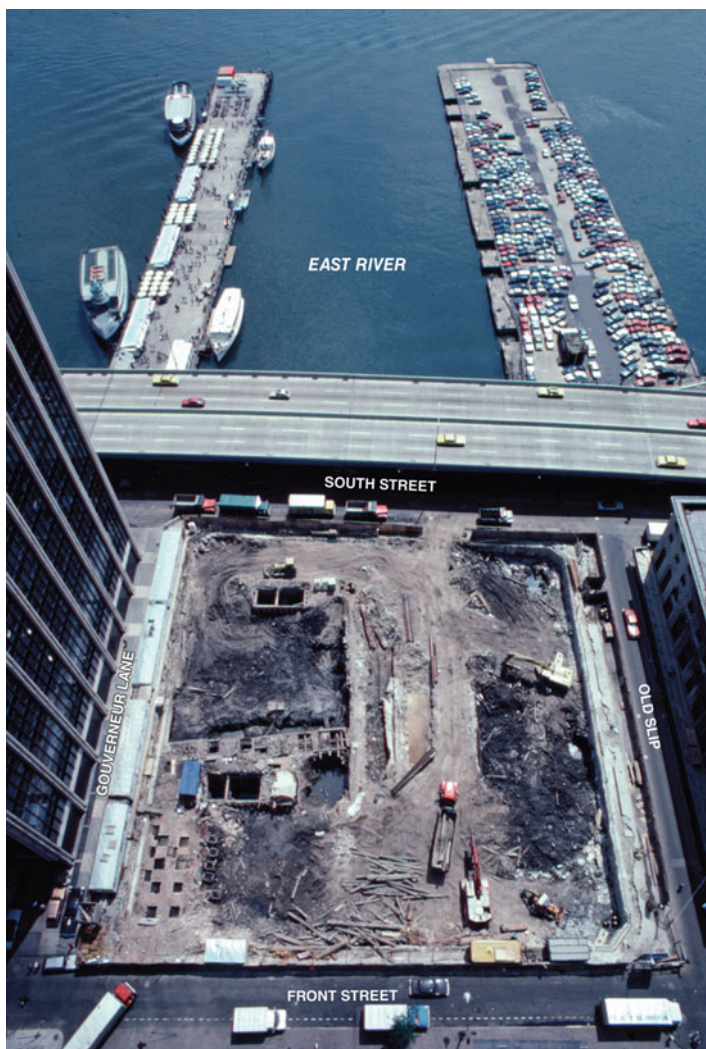
Fig. 19.2 Aerial view of the Assay site showing 5' x 5' units placed in a checkerboard pattern in Lot 9, Anthony V. Winans lot (Louis Berger & Associates 1990, Courtesy New York State Museum, Albany, NY)
