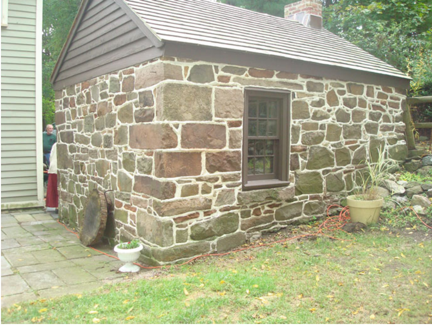
Fig. 5.2 Extant Eighteenth-Century Bakehouse/Out Kitchen (the John H. Vreeland Out Kitchen, Towaco, Morris County, NJ. HABS NJ 493; Photograph by Elena J. Fletcher)
