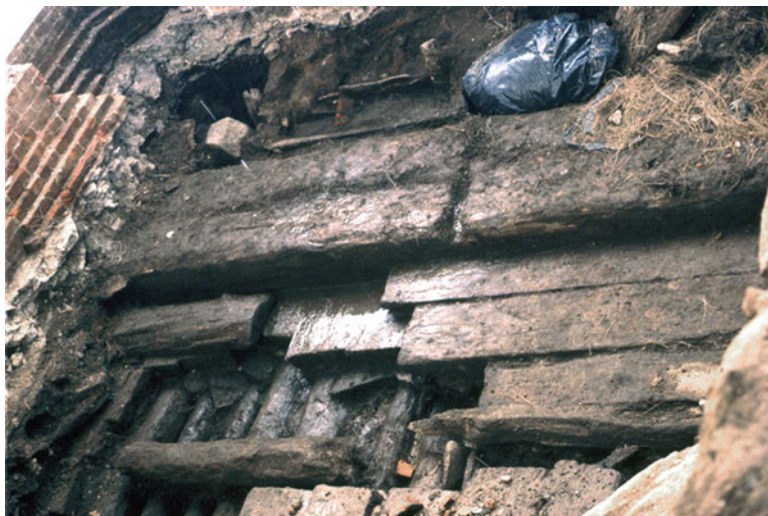
Fig. 7.6 Spread footers (thick wood planks) straddling the western edge of the landfill and the eastern edge of the exposed logs of the wharf/grillage created by the mid-eighteenth-century water lot grantees, among them Ann Elizabeth Staats Schuyler. (Photo by Drew Pritzger in the author's collection)
