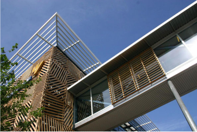
Fig. 32.1 Detail of the university building facade. Source: Collection Windesheim University
