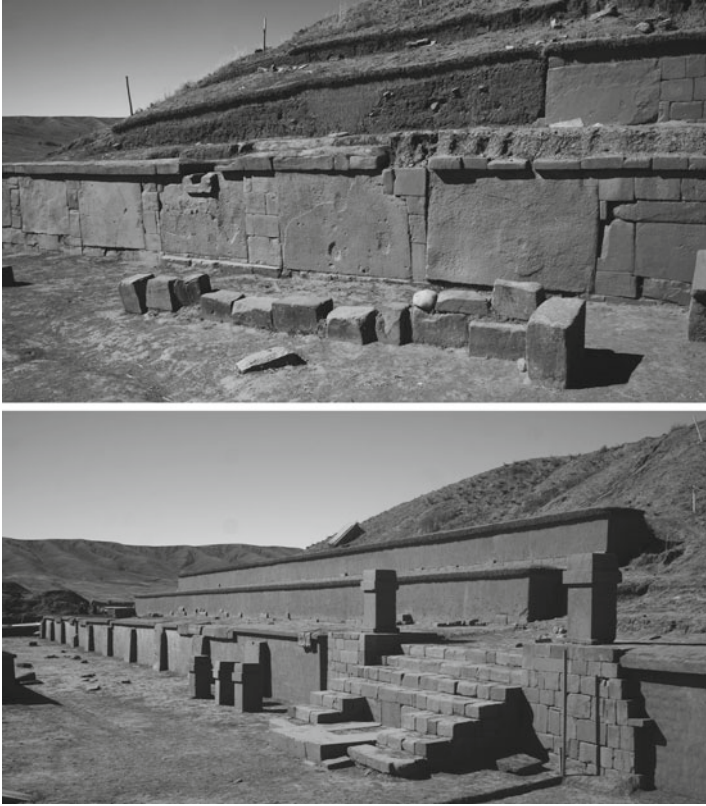
Fig. 4.5 The west or “front face” of the Akapana, highlighting the strategic placement of andesite veneer pilasters in a sandstone terrace foundation. Andesite constitutes the large rectangular blocks in the upper image , which depicts the inset north “wing” of the second terrace west façade, and the intermittent pilasters in the lower image . Note: the sandstone facing of the west lower terrace facade in the lower image has been covered with mud facing for purposes of conservation) (photos by J. Janusek)
