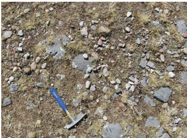
Fig. 3.6 Road surface in the Inca section of the Huaccoto quarry, with surfacing of small pebbles
