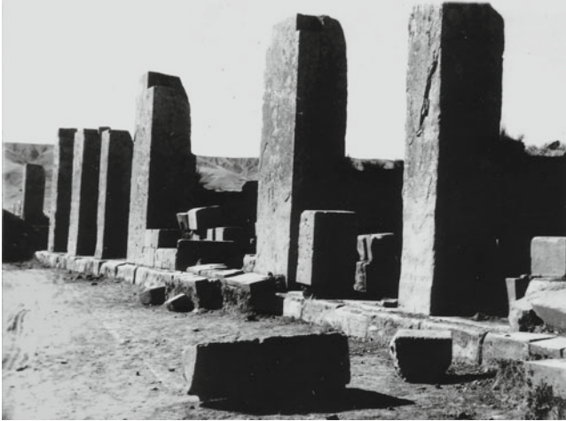
Fig. 4.8 Kalasasaya's West Platform and balcony wall, prior to their reconstruction (photo by Gregorio Cordero Miranda, courtesy of Alexei Vranich)
