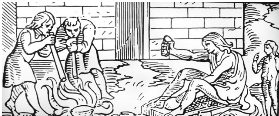
Fig. 10.2 Benzoni woodcut showing sopletes in use with a crucible
