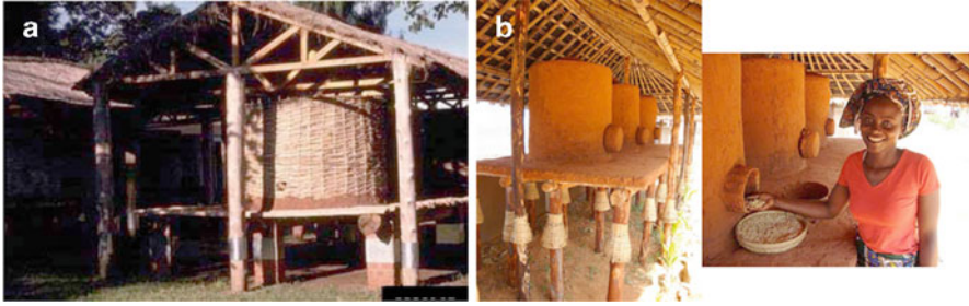
Fig. 8.6 Examples in developing countries of innovative, inexpensive structures for short-term storage of seeds, for consumption and for replanting. (a) Container for field corn grain in Malawi. The storage structure is raised above ground to avoid rodent infection and flooding, and shelter is provided to minimize exposure to the sun. Courtesy of H. F. Schwartz, Colorado State Univ., http://www.bugwood.org . (b) Woven bamboo storage silo, Mozambique, covered with clay, with caps to cover the openings for filling and emptying. It stands on a base that incorporates vermin traps and under a simple shelter to maintain cool, dry, and even conditions. Courtesy of HELVETAS Swiss Intercooperation. http://www.flickr.com/photos/44345799@N05
