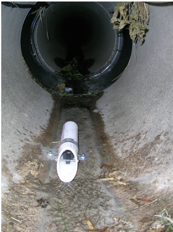
Fig. 10.2 Installation of a temperature probe in a sewer pipe
