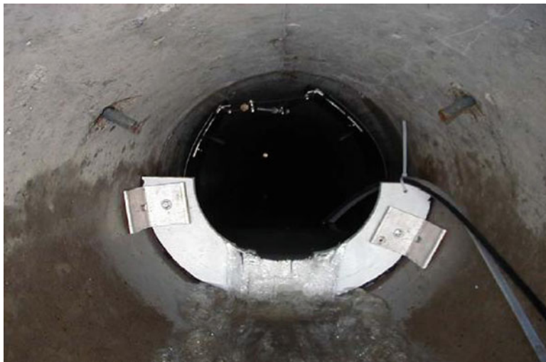
Fig. 8.5 Circular weir installed in the outlet pipe of the pond
