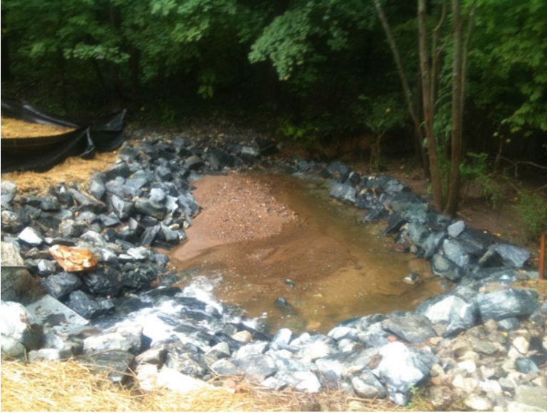
Fig. 5.15 Sedimentation downstream of a stormwater treatment practice indicates a potential malfunction (©Stormwater Maintenance, LLC, www.SWMaintenance.com , reprinted with permission)
