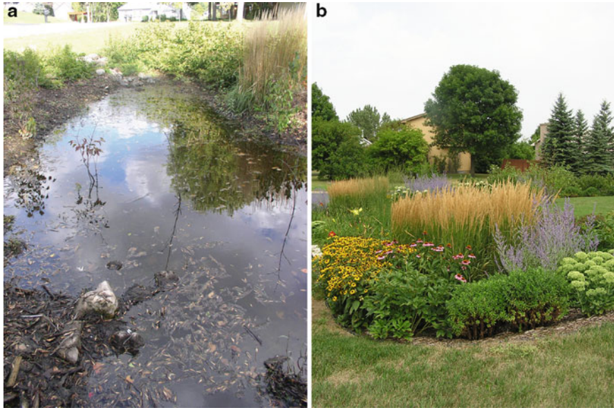
Fig. 5.1 Examples of visual inspection for a rain garden that is not functioning properly ( left ) and a rain garden that may be operating properly ( right ) (Photos by B. Asleson)
