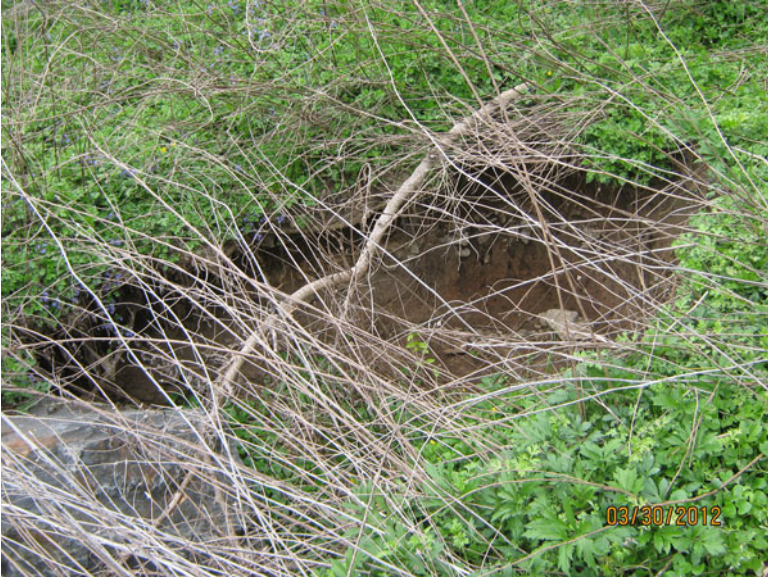
Fig. 5.8 A channel that exhibits signs of erosion through bare soil and a fallen tree (©Stormwater Maintenance, LLC, www.SWMaintenance.com , reprinted with permission)
