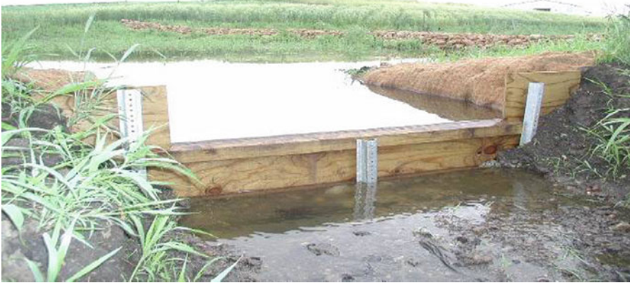
Fig. 8.4 Rectangular weir at the inlet of the pond, which was later modified
