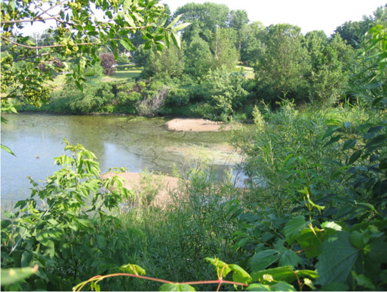
Fig. 5.14 Sediment deposition in a retention pond (©John Chapman, reprinted with permission)
