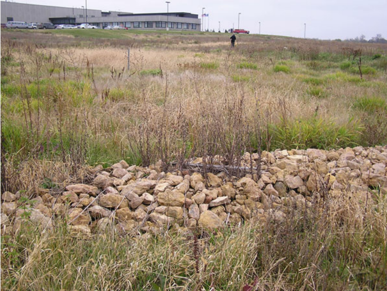
Fig. 4.8 Soil filter at Carver County maintenance facility, Minnesota, with permeable overflow weir in the foreground
