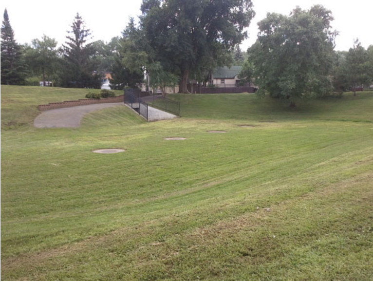
Fig. 4.1 Example of a dry pond
