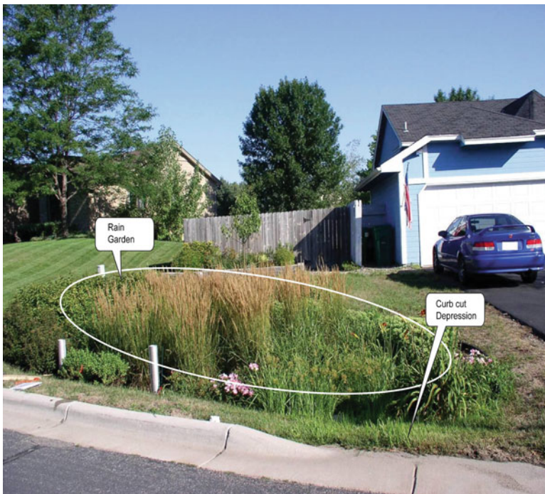
Fig. 4.13 Example of a curb cut out that allows road runoff to enter a rain garden
