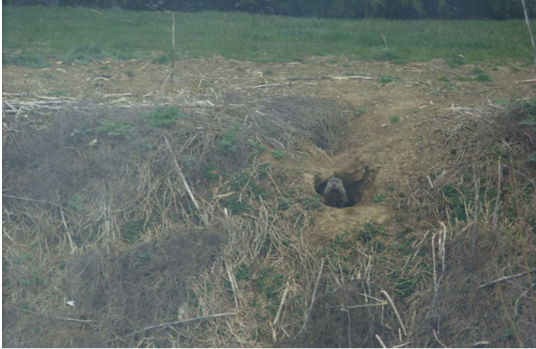
Fig. 5.13 A groundhog and burrow within a stormwater treatment practice (©Stormwater Maintenance, LLC, www.SWMaintenance.com , reprinted with permission)
