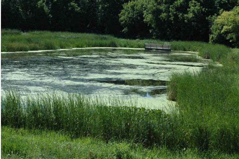
Fig. 4.2 Example of a wet pond
