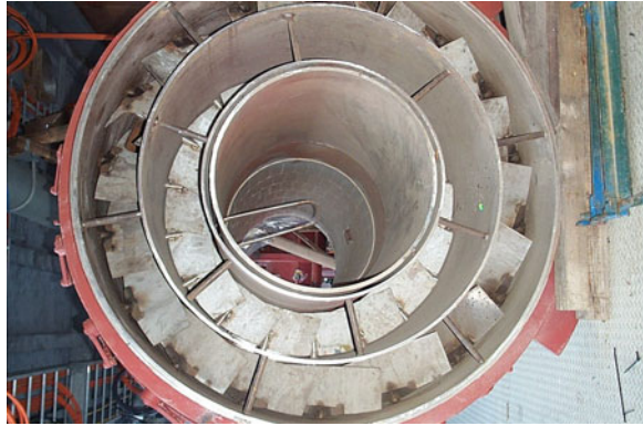
Fig. 11.10 A pf burner nozzle seen from the furnace (Courtesy of Millmerran Operating Company, Australia)
