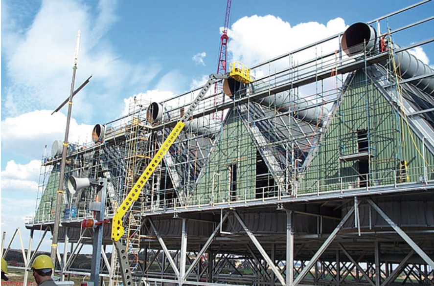
Fig. 15.4 A large ACC during construction (courtesy of Millmerran Operating Company, Australia)
