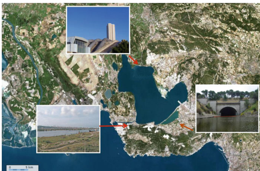
Fig. 1 Aerial view of the Berre Lagoon (southern France). The three superimposed images are of the Saint Chamas hydroelectric plant ( top ), the Rove tunnel ( right ), and the Caronte channel ( lower left ). See text for explanation ( source : Géoportail 2011)
