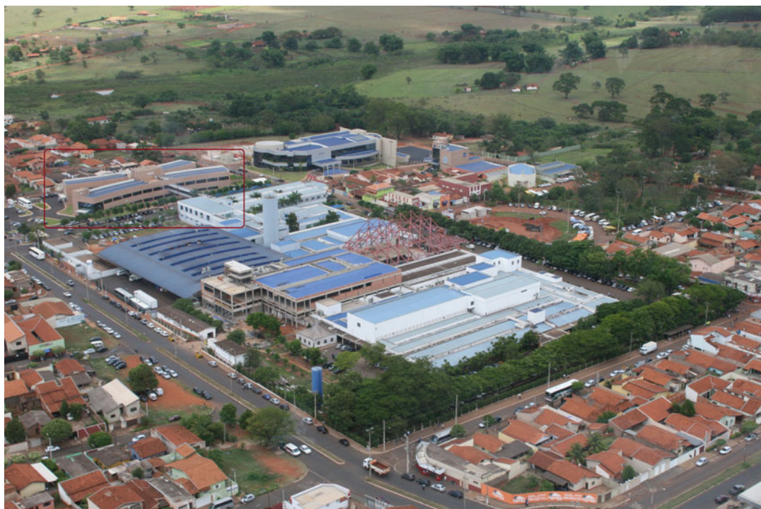
Fig. 10.12 Barretos Cancer Hospital complex. The red rectangle highlights the Cancer Prevention building that also includes areas for molecular oncology investigation, blood transfusion, and an Institute of Education with graduate courses in oncology
