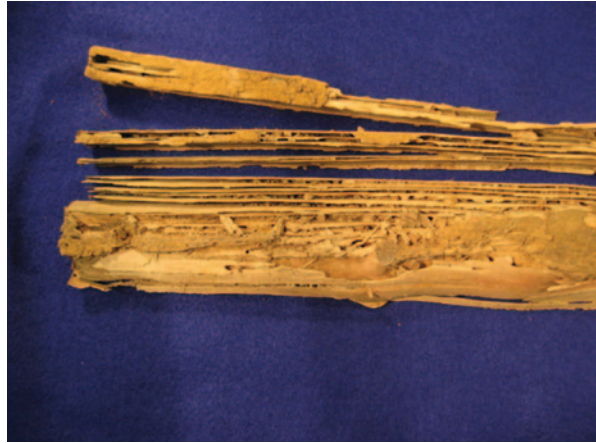
Fig. 12.2 Subterranean termite damage to a 2.5 \times 10 cm ( 1 \times 4 in.) board
