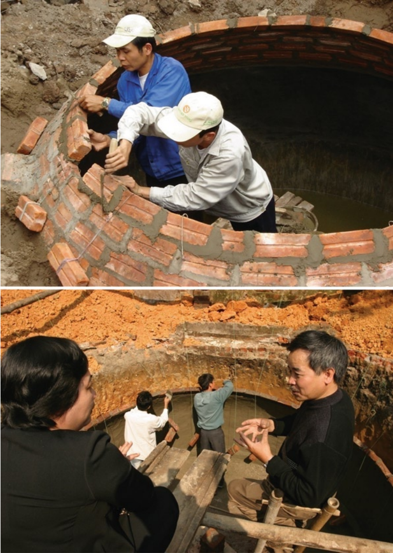
Fig. 2.3 Biogas plants being put up in Vietnam (photo courtesy: SNV, Netherland Development Organization)
