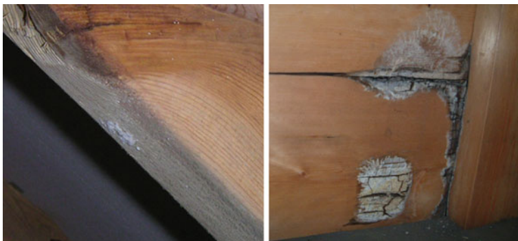
Fig. 14.49 Wood decay in incipient stage ( left ) and progressed stage ( right ) featured by hyphae
