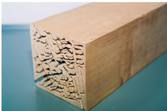
Fig. 14.53 Wood attacked by termites
