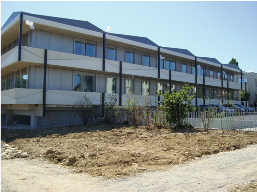
Fig. 16 North-east façade of IUCN headquarter building
