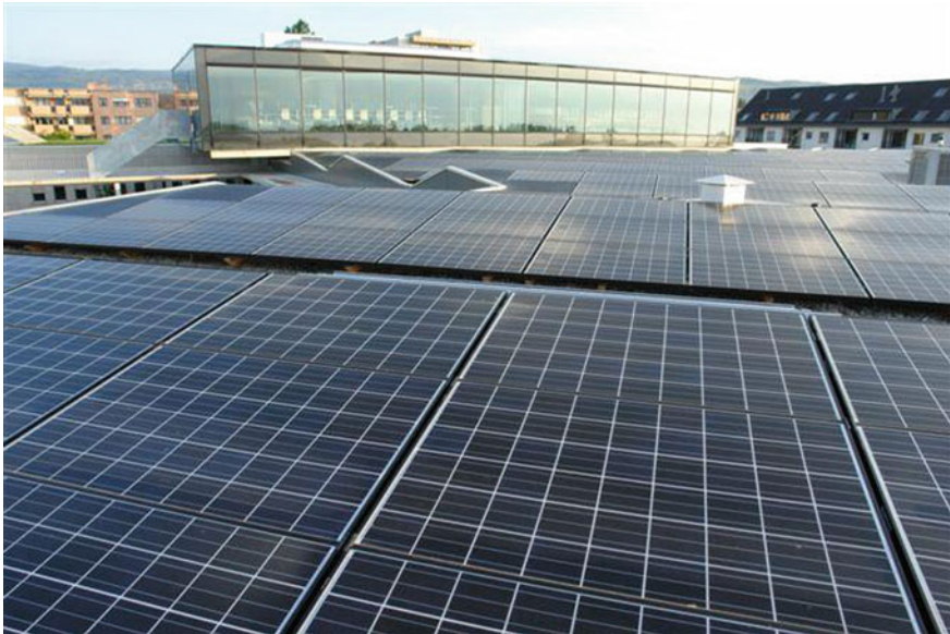
Fig. 18 PV installation on the roof
