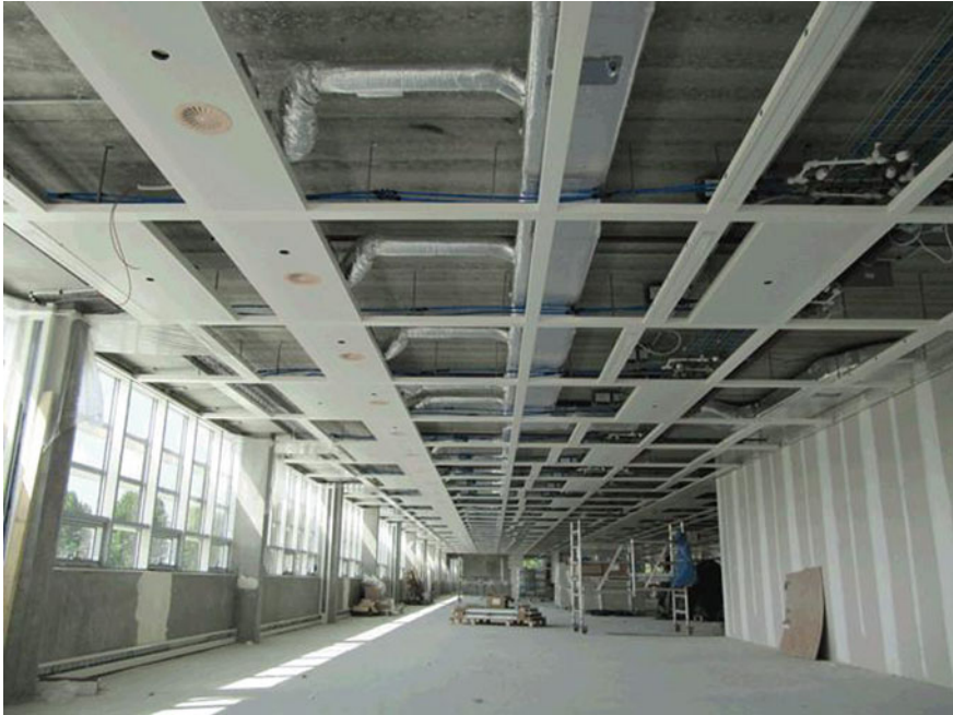
Fig. 25 Ceiling panels for heating and cooling with integrated air diffusers
