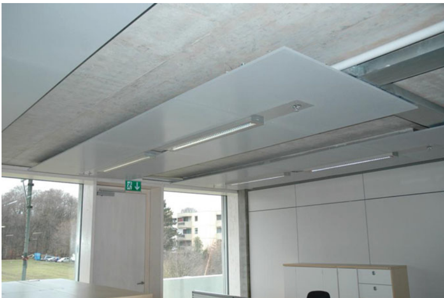
Fig. 19 Ceiling panel for heating and cooling, with integrated extract air terminal and lighting
