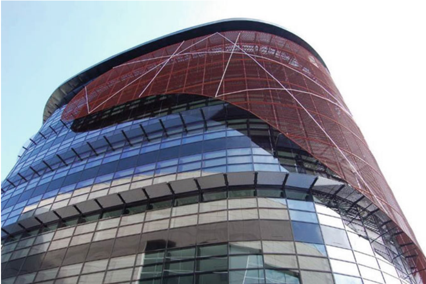
Fig. 3 Solar shading of the facade
