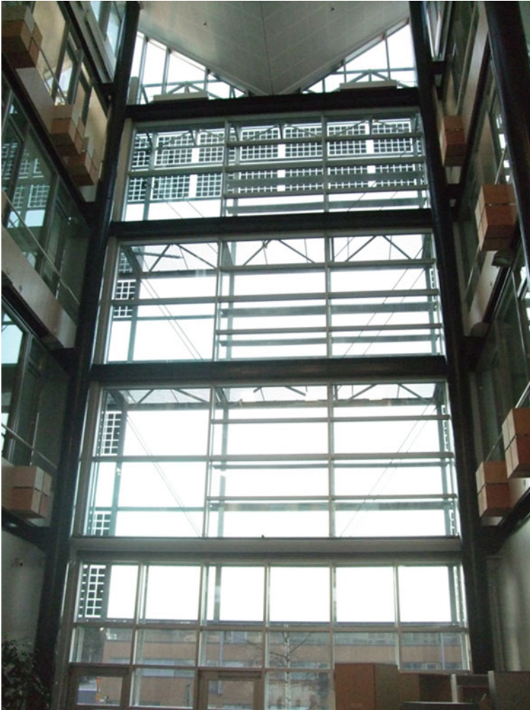
Fig. 11 Atrium space of the building has no installed cooling and overheating is avoided by opening bottom and top windows. Motorized openable windows are to be open manually when needed and will be closed by weather station control (wind, rain, and temperature control) automatically
