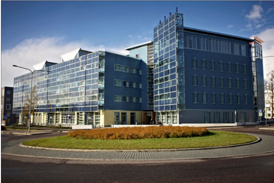
Fig. 9 Ympäristötalo in Helsinki, Finland. South facades are double skin facades with integrated PV. All façade are different because of daylight and solar shading considerations. Photograph Mari Thorin, Rhinoceros Oy
