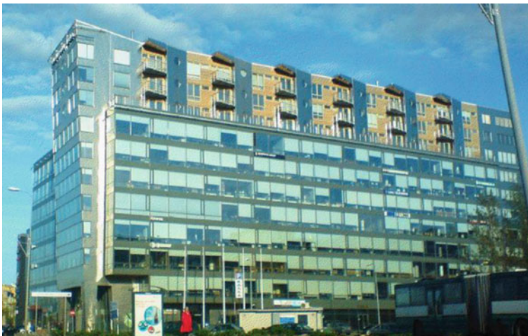
Fig. 16 Solar shading of the facade is not resolved. Most of curtains are constantly closed. During daytime, spaces are lighted with artificial lighting, instead of daylight
