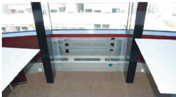
Fig. 5 In the mixed mode operation, façade intakes and low-pressure atrium exhaust fans are used. This is used for the night-time ventilative cooling and, in the midseason, when the ventilation by air handling units is forced for cooling purposes
