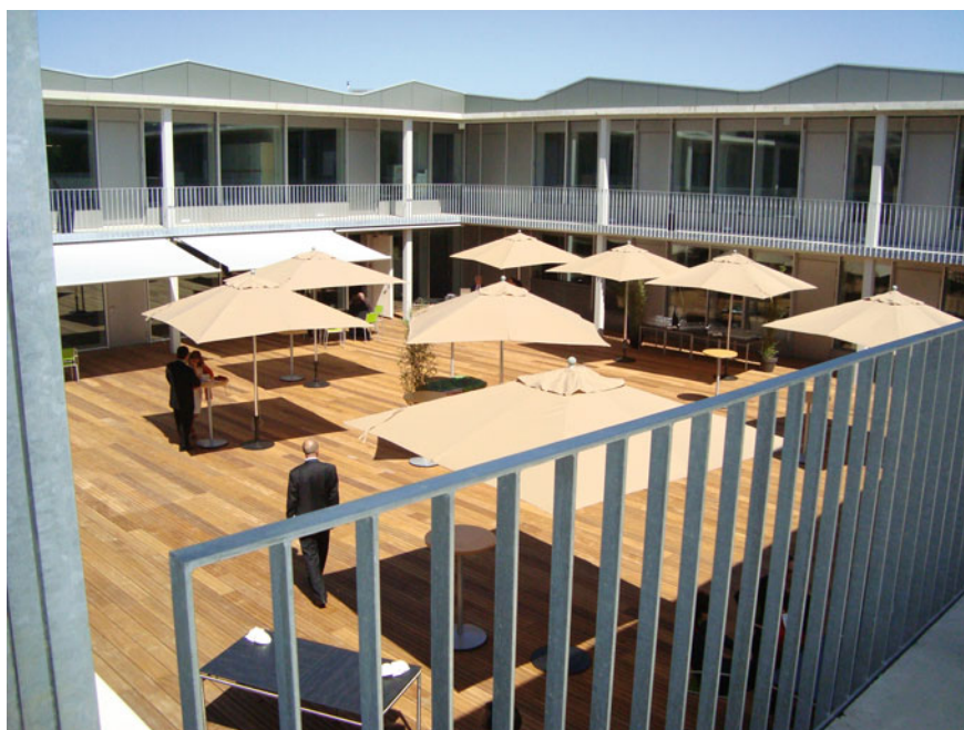
Fig. 17 Inner courtyard of the building
