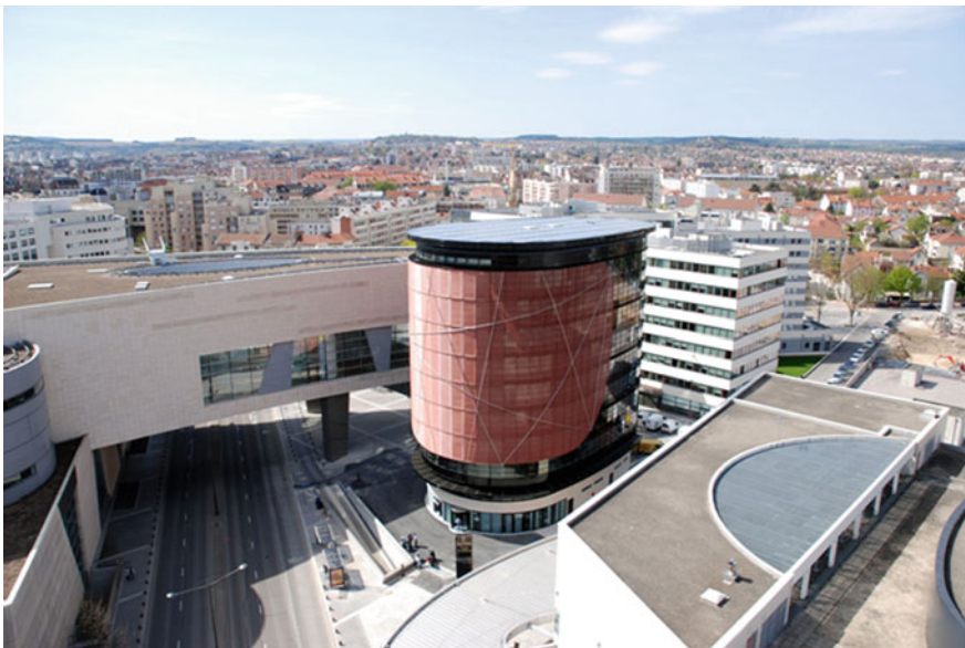
Fig. 1 Elithis Tower in Dijon, France
