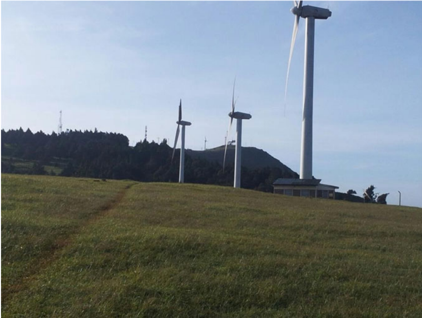
Fig. 2 Wind turbines facing the top of Ngong Hills. What is not visible is the new power substation, which is situated after the third wind turbine
