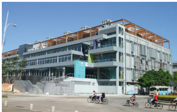
Fig. 15 The tested office building in Shenzhen
