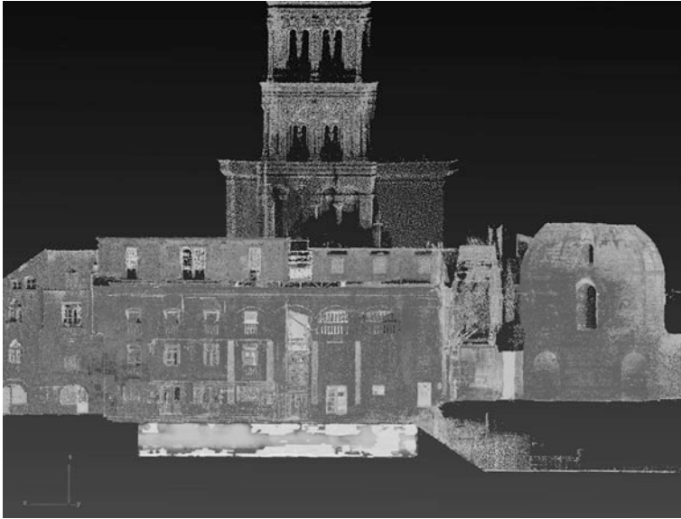
Fig. 6.16 Model combining GPR and laser scan point cloud data. The viewpoint is from west of the western façade of the Peristyle (courtesy of Central Dalmatian Archaeological Project)
