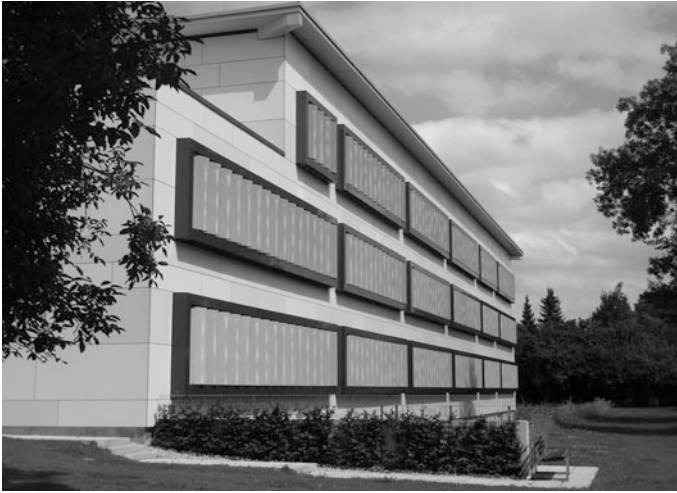
Fig. 20 View of a refurbished school using VIP for the insulation of the base slab
