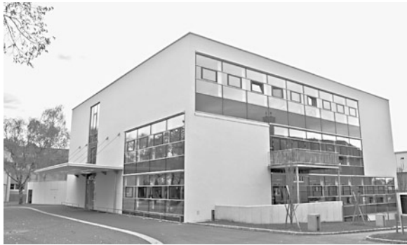
Fig. 8 Sonderschule 6: a compact shape and large windows for increased daylight. Shading is provided by screens rolled up in slim casings Photo Xavier Dequaire
