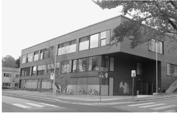
Fig. 5 Sonderschule 4: a new storey provides additional space preserving a compact shape. Large windows increase daylight. Venetian blinds provide shading. The original columns are included into the thermal envelope. Photo Xavier Dequaire
