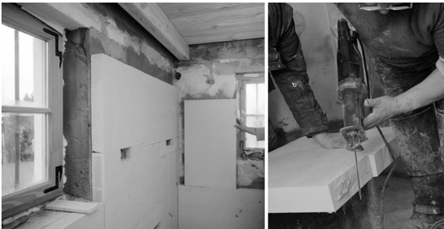
Fig. 28 Installation of the interior thermal insulation with CALOSTAT ® in combination with a calcium silicate insulation material ( left picture ). Right picture The calcium silicate board with microporous insulation kernel, i.e. CALOSTAT ® , allows a time and cost-efficient installation and an individual adjustment at the construction site
