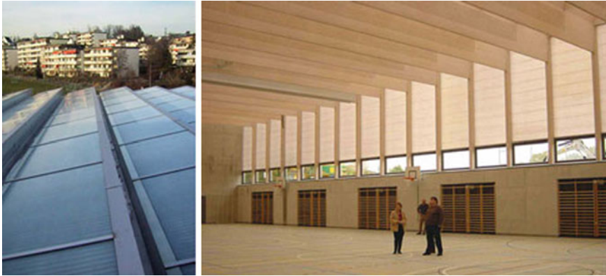
Fig. 9 The school Buchwiesen in Zurich: example of the use of granular-aerogel-filled Scobatherm glass fibre composite panels in the form of a transparent daylighting roof (2003)
