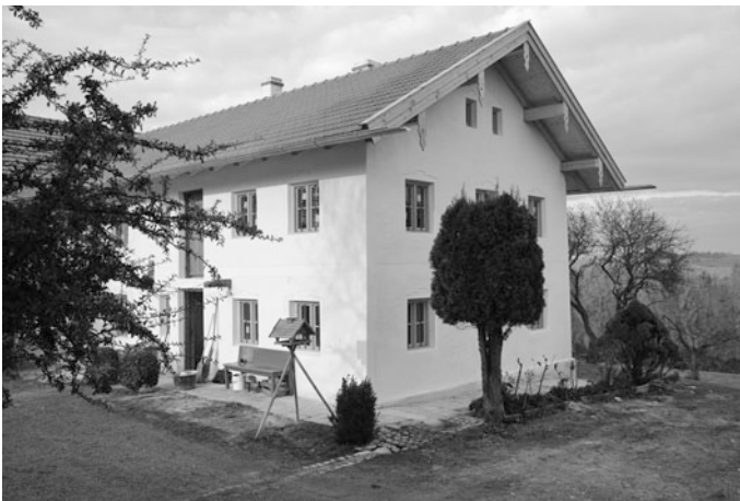
Fig. 26 Prospect of the farm house which was refurbished by using an internal thermal insulation to keep the historical identity of the building
