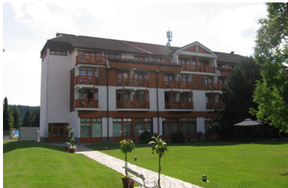
Fig. 3.51 A six-storey Hotel Dobrava in Terme Zreče, the Pohorje Mountain, Slovenia
