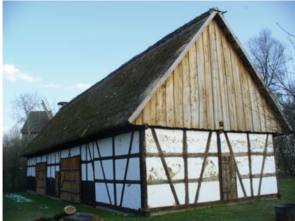
Fig. 3.26 Rural types of old timber-frame construction with a visible load-bearing frame
