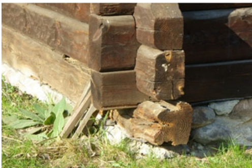
Fig. 3.18 Types of connections in log construction; (a) the old type, (b) the new type
