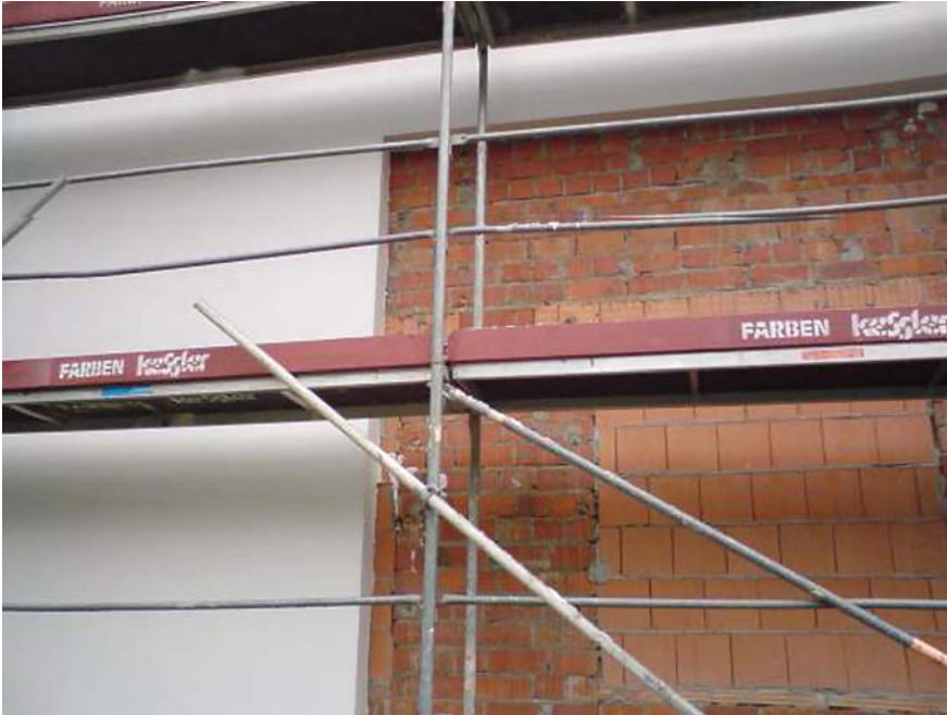
Fig. 4.2 A commonly used insulation material in walls, roof and basement ceiling is Styropor® (BASF), similar to polystyrene
