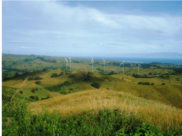
Fig. 5 Butoni wind farm in Fiji
