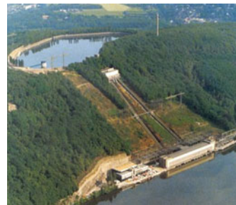
PHS facility at Alaska [14]
