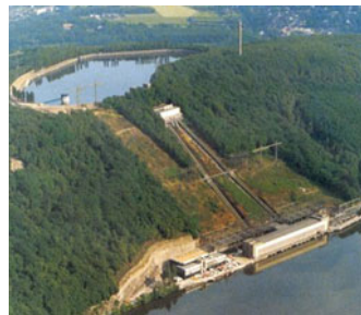
PHS facility at Alaska [14]
