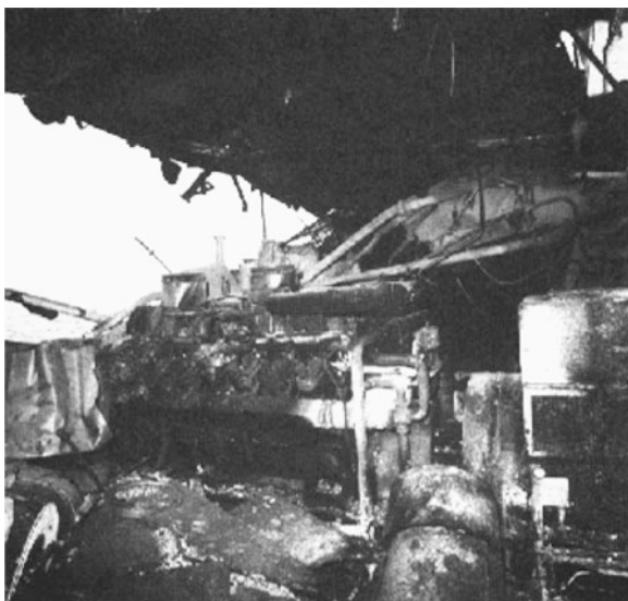
Fig. 4.1 Engine room on west Vanguard after explosion, looking out to sea
