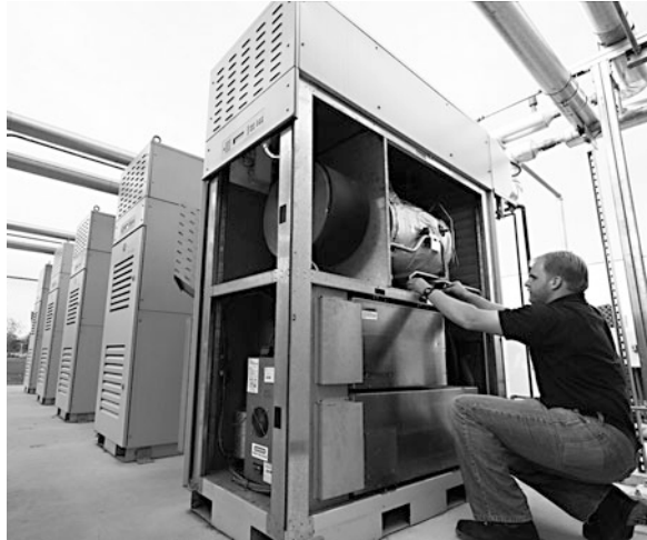
Fig. 8.1 Installation of several 65 kW microturbines
