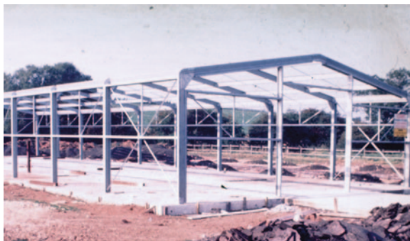
Fig. 1.2 Cold-formed steel portal framing system
