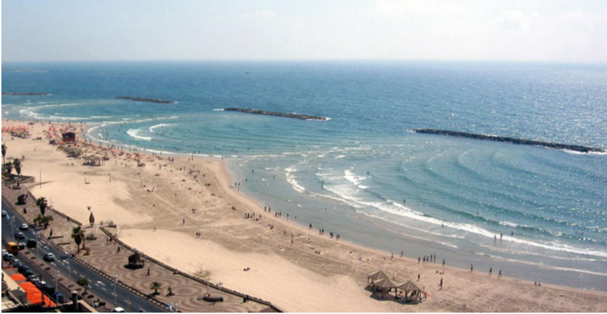
Fig. 19.6 Image of water waves interacting with a breakwater taken from Ref. [5]
