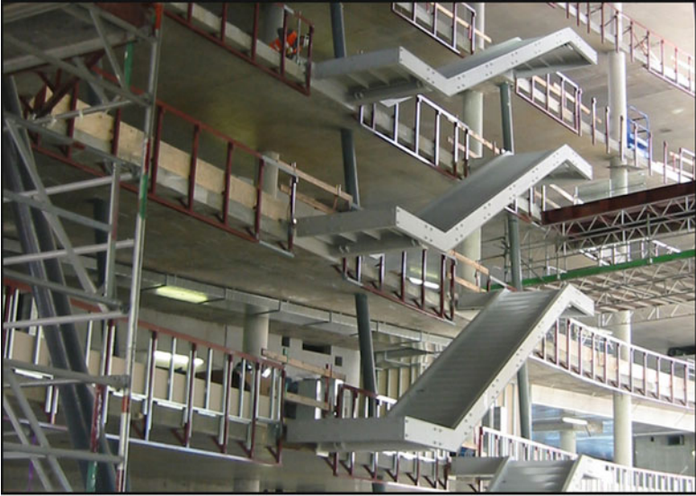
Fig. 4.12 Inside the domicile building under construction
