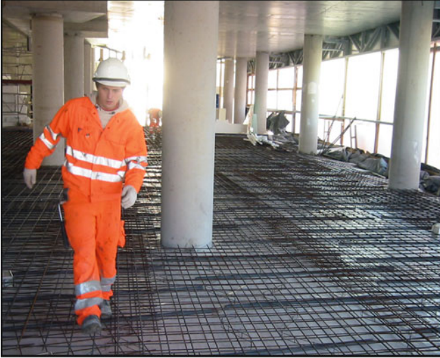
Fig. 4.10 Engineer passing the load bearing columns
