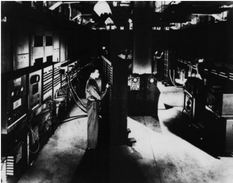
Fig. 3.6 Setting the switches on ENIAC's function tables (US Army photo)
