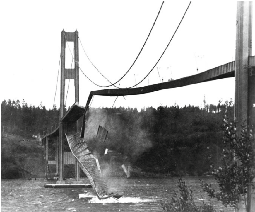
Fig.1.2 A cautionary tale and textbook example of severe resonance effects: the collapse of the Tacoma Narrows Bridge due to wind induced aeroelastic flutter and the resulting resonance [25]
