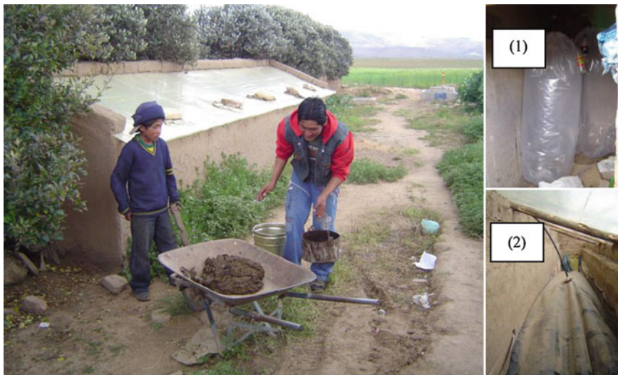
Fig. 6 Biogas digester in the Altiplano, 4,100 m above mean sea level; gas tank (1), digester (2)
