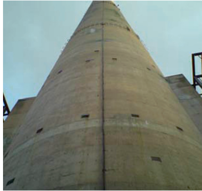
Figure 2: Flue ducts flanking chimney on the bottom.
