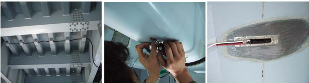
Fig.3 Sensor attachment on the deck plate of bridge
