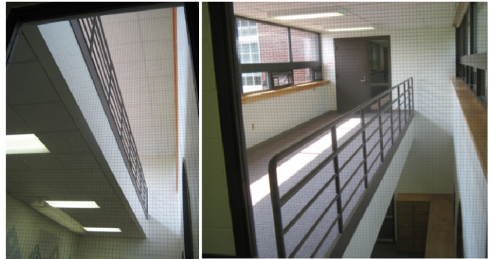
Figure 2: (a) View of underside of the bridge (b) View from top of the bridge
