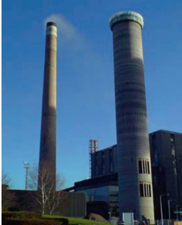
Figure 1: The old chimney without TMD on the left; the FGD chimney is on the right.
