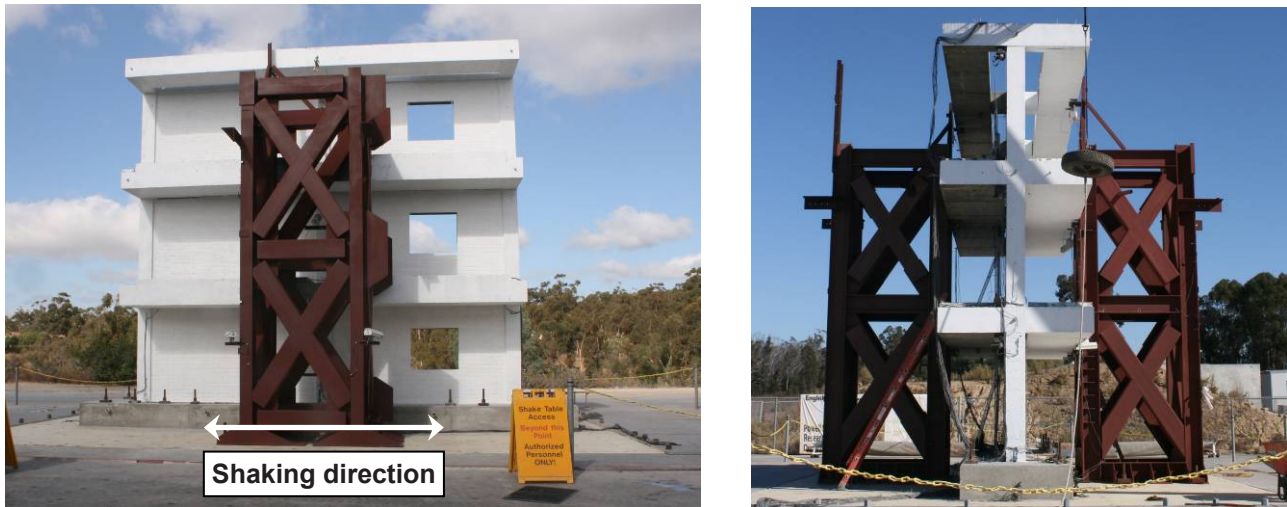
Fig. 2 Front view (left) and side view of the specimen (right)
