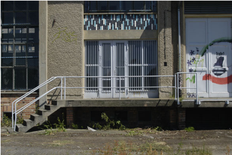
Fig. 14.12 Entrance to an electrical transformer and plant building
