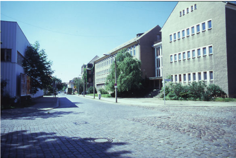
Fig. 14.10 Freienwalder Strasse looking away from the prison towards the main entrance to the complex. To the left is the communications facility and to the right the offices of the chemistry service and criminal technical institute
