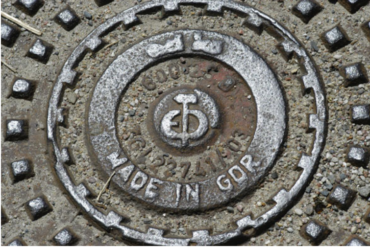
Fig. 14.11 Manhole cover, made in the GDR
