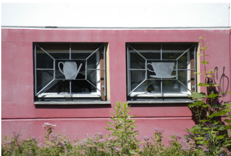
Fig. 14.4 Barred windows of the main canteen on Gensler Strasse
