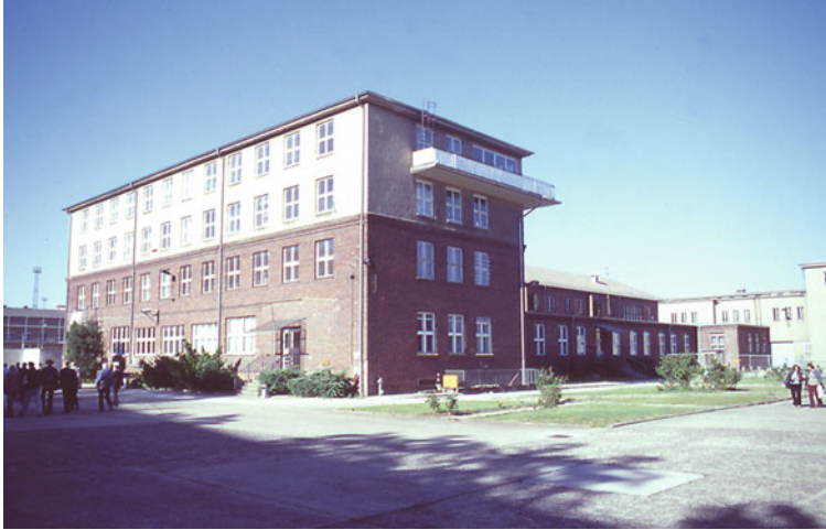
Fig. 14.15 The main prison building. The lower brick portion represents the 1930s National Socialist communal kitchen; post-war it was raised in height
