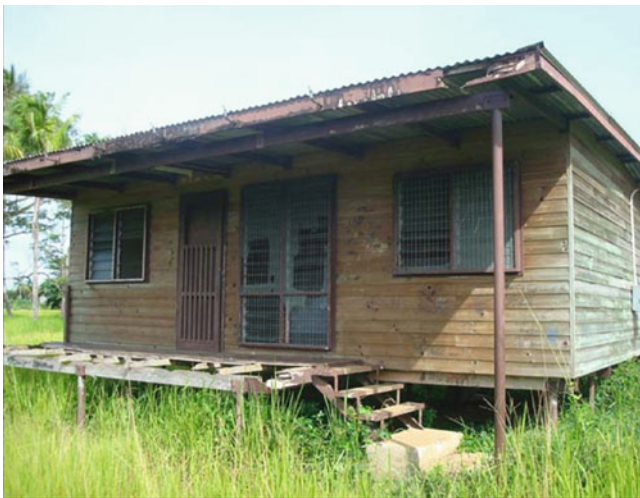
Fig. 12.11 Closed Nomad sub-district office building, 2008. (Photo credit: Bruce Knauff)
