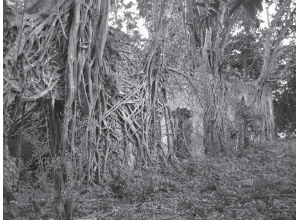
Fig. 5.1 Front wall of Mgoli in 2004
